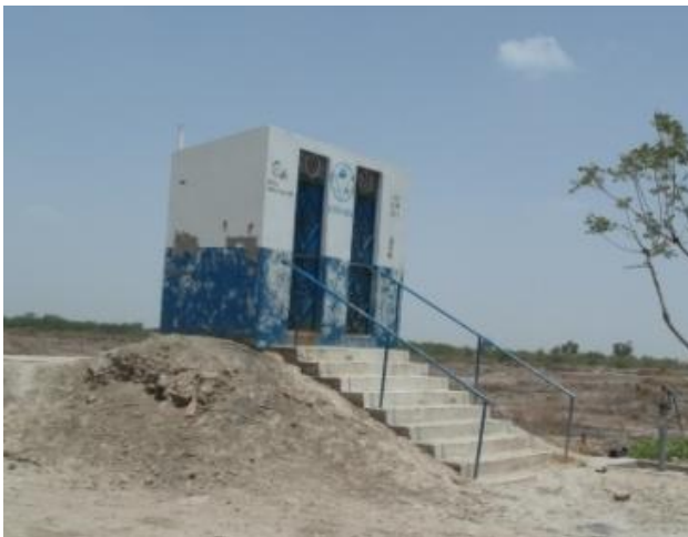
Toilet on higher ground
