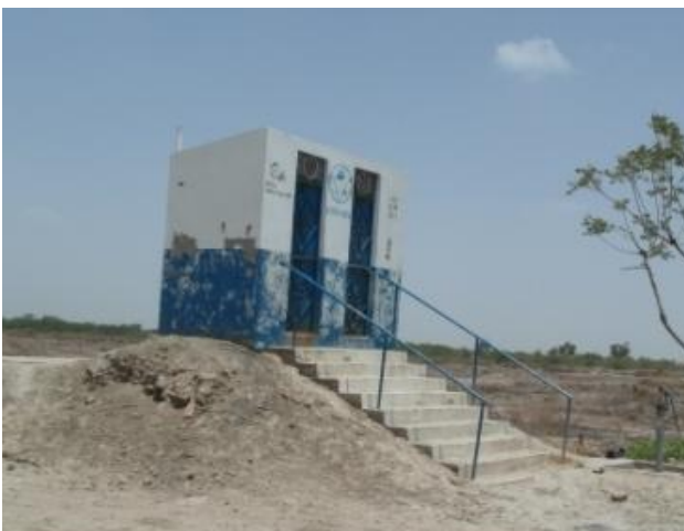
Toilet on higher ground
