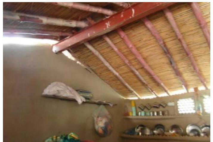
House built with bamboo
