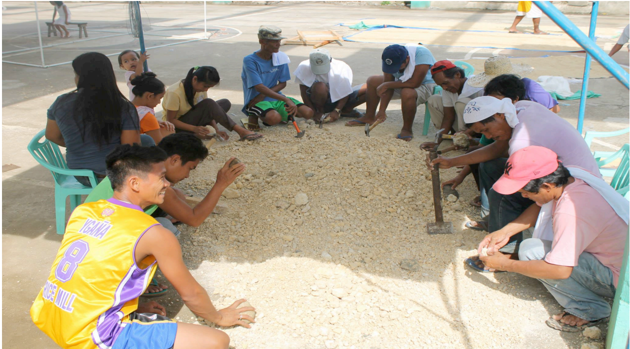
Figure 1 Preparing earth for the Interlocking Compressed Earth Block [ICEB]
